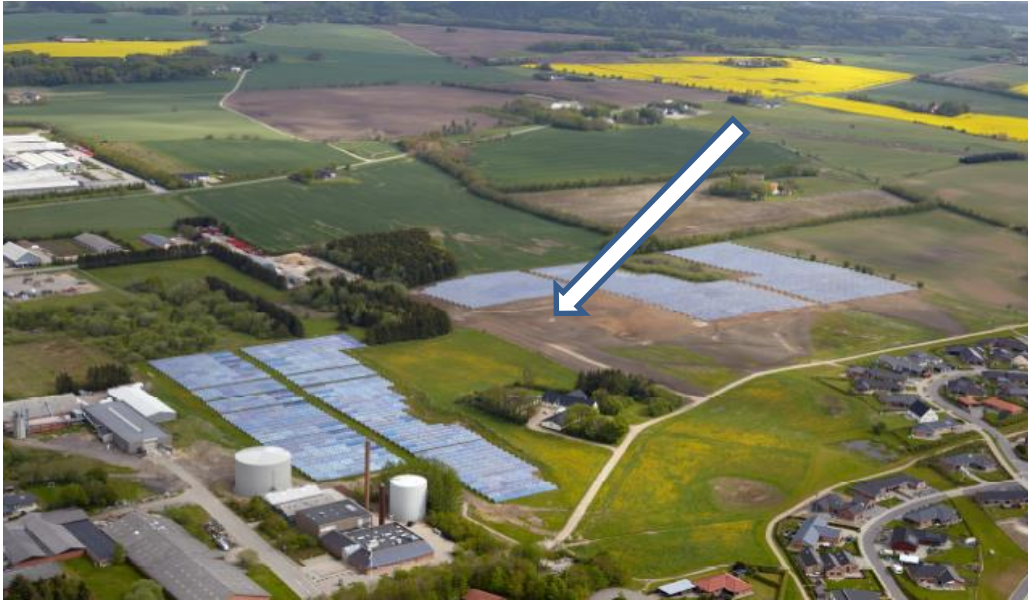
Figure 46: Borehole thermal energy storage of the solar district heating plant in Brædstrup, Denmark (Source: PlanEnergi)
