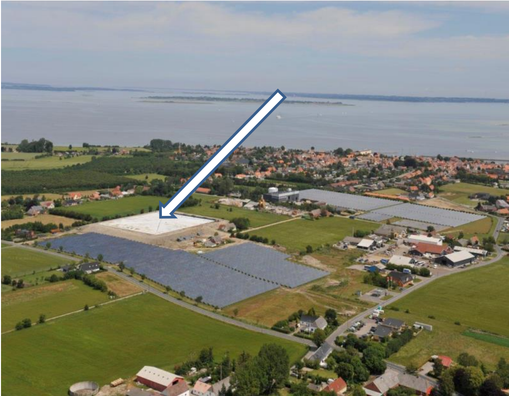
Figure 44: Pit thermal energy storage in Marstal, Denmark (Source: PlanEnergi)
