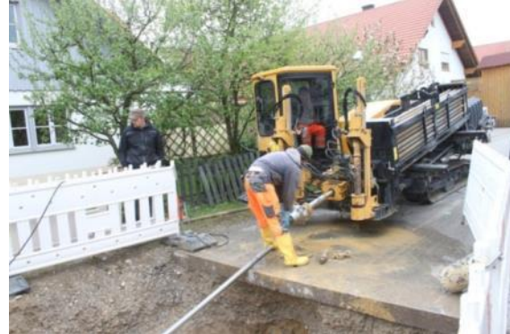
Figure 53: Directional drilling machine (Source: Rutz)
