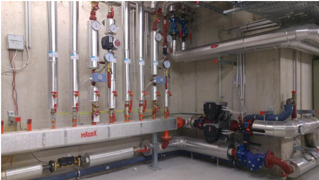
Figure 58: Heat distribution at a business building with DH supply (Source: Güssing Energy Technologies)
