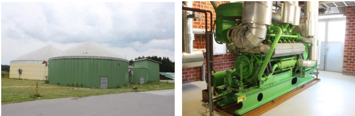
Figure 23: Digesters of an agricultural biogas plant (left) and CHP unit (right) of a biogas plant (Source: Rutz D.)
