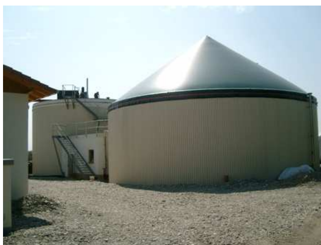
Figure 4.7 Vertical digester in Germany, built in 2005 for digestion of energy crops (KRIEG and FISHER 2008)
