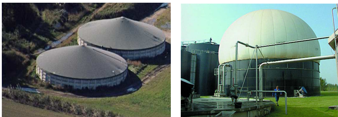
Figure 7.33 Membrane covered storage tanks (DANISH BIOGAS ASSOCIATION 2008)
