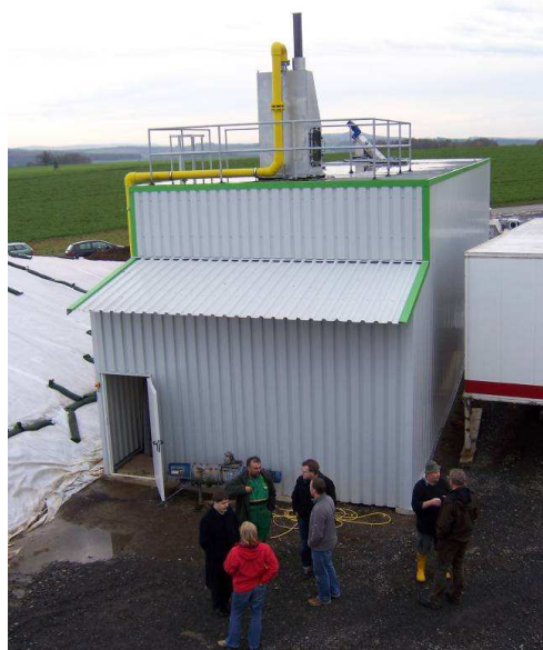
Figure 7.21 Horizontal plug-flow digester (RUTZ 2006)
