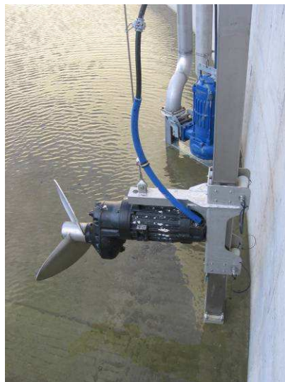
Figure 7.22 Submersible motor propeller stirrer (AGRINZ 2006)
