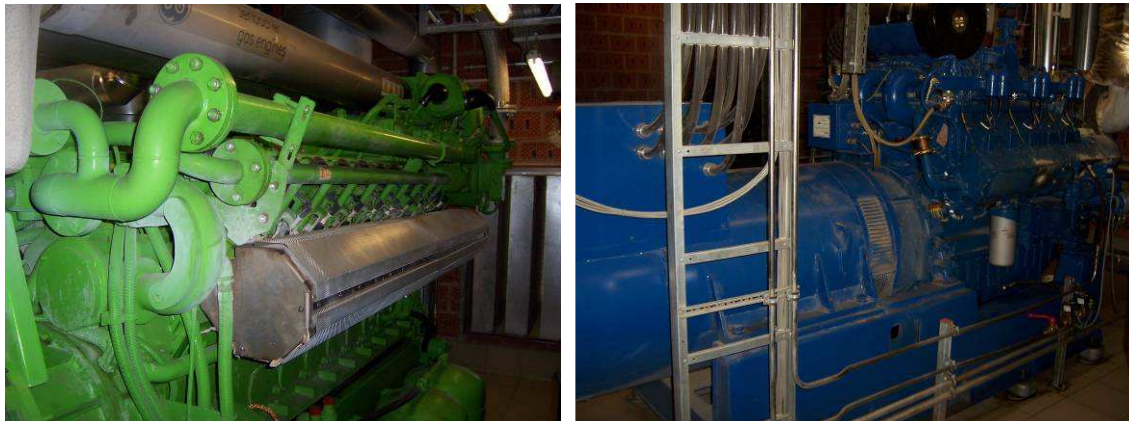
Figure 5.3 Gas-Otto engines (RUTZ 2007)
