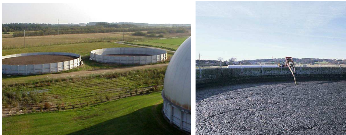
Figure 7.32 Storage tanks covered with natural floating layer (DANISH BIOGAS ASSOCIATION 2008)
