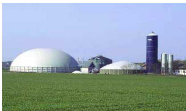
Figure 4.5 Picture of farm scale biogas plant in Denmark, co-digesting animal slurries and energy crops (GROENGAS A/S)
