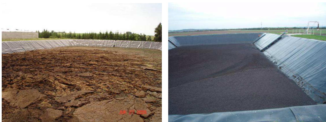
Figure 7.34 Open pond lagoons for digestate storage (AGRINZ 2006)
