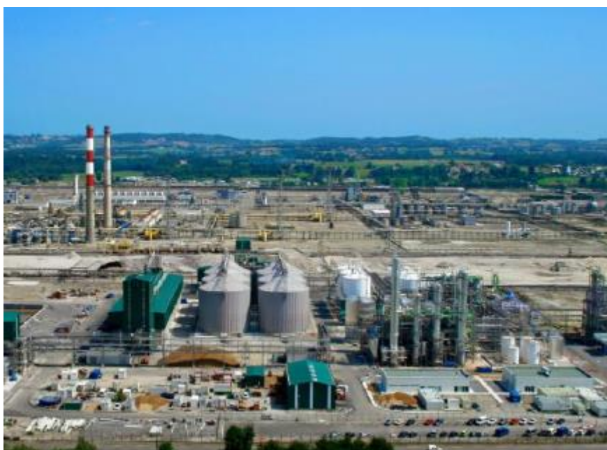
Figure 46: Abengoa Arance EC demonstration plant, France (Abengoa Bioenergy Annual Report 2010)
