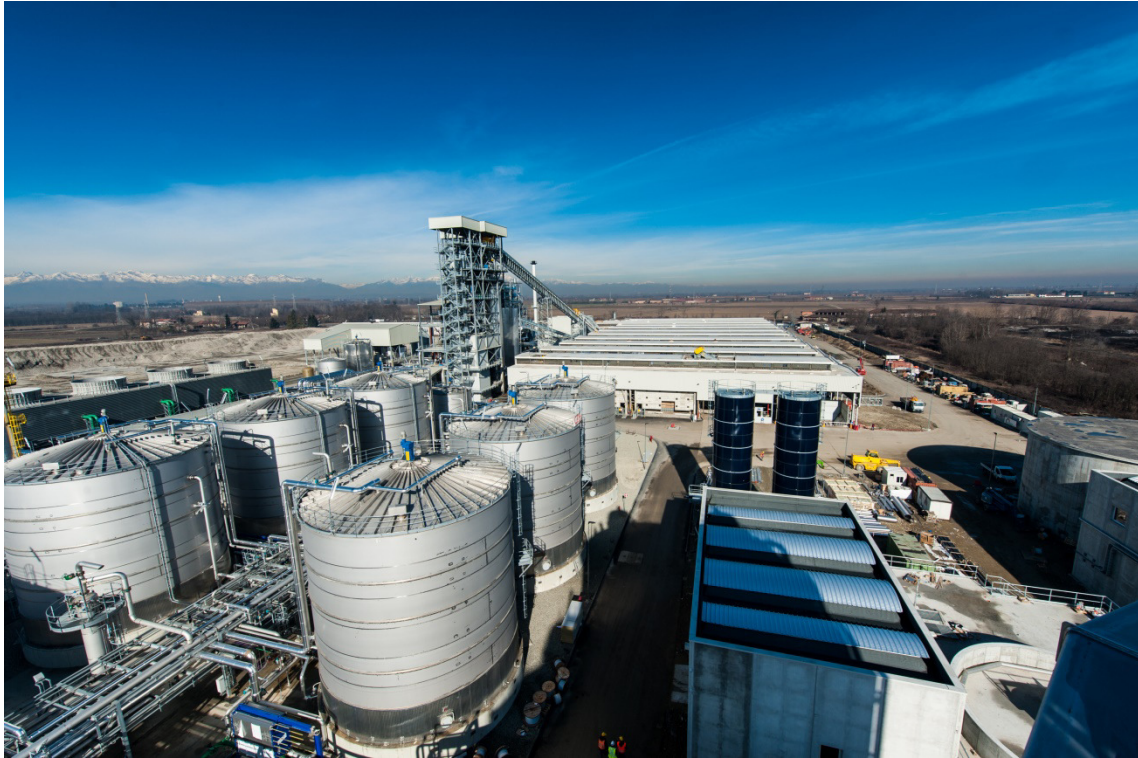
Figure 4: Aerial view of the Crescentino ethanol plant
