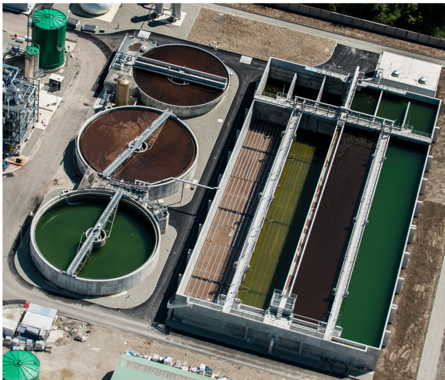
Figure 33: Waste water treatment area
