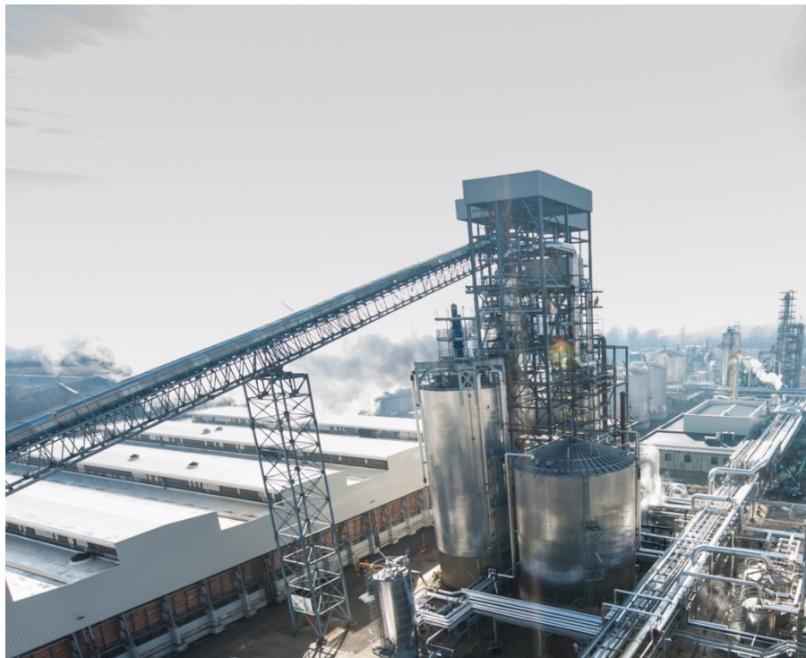
Figure 16: The pretreatment area with the biomass feeding system
