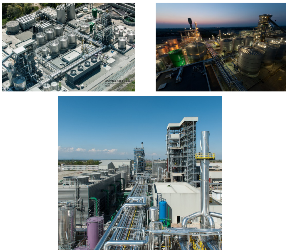
Figure 8: Plant constructed at present day
