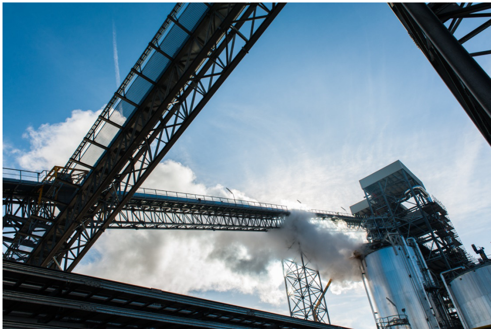
Figure 20: The pretreatment area
